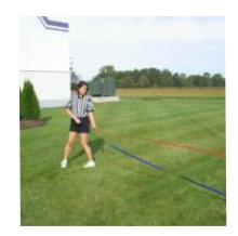
NOW, Project accurate cross lines by attaching a string line to the corner spike, pulling it across the field, keeping the line directly (o/c) above the length of the Blue guide...
