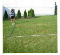
2) Establish your 1st corner location on the Base Line by spiking down the ends of the WHITE & BLUE guides directly (On Center) under the string line...
